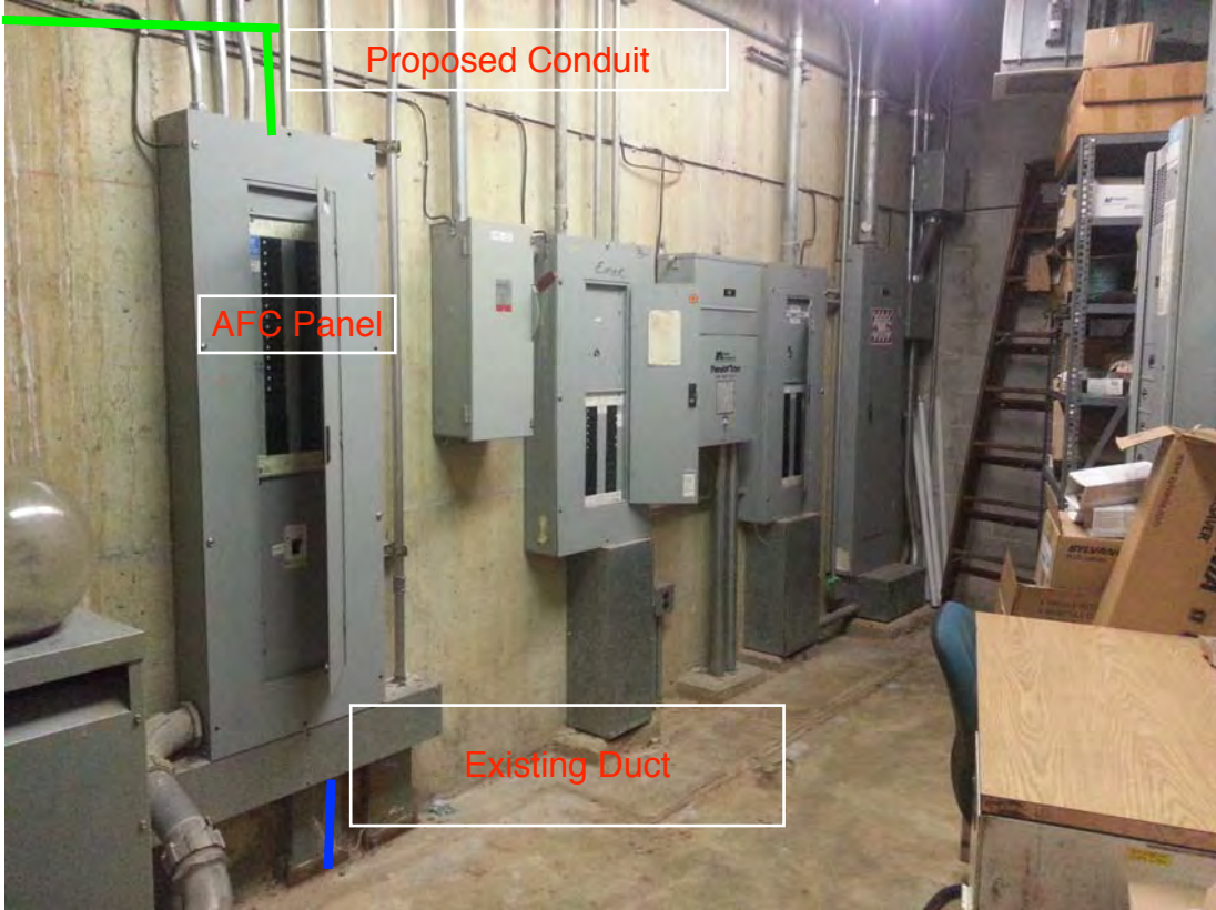
Photo #5 – Existing and Proposed Route in Room C106
